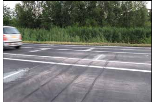
Intercomp sensors installed in staggered pairs in each traffic lane.
