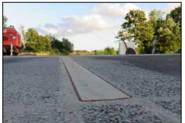
Intercomp strip sensors are grouted in place and ground flush with the pavement.
