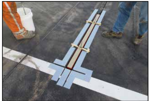
Sensors are installed into channels cut into pavement.
